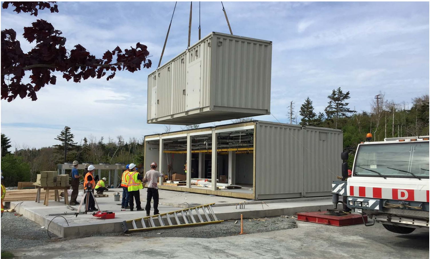
Installation of Vertiv™ SmartMod™
